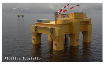
During the feed-stage the project considered using a subsea substation. This would remove the need for a lot of dynamic cables but would change the installation methodology as well as maintenance. The project was optimistic but concluded that the technology was not yet ready and decided to go for a floating substation instead.
